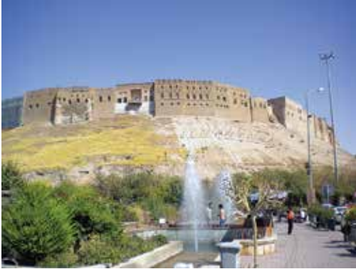
Figure 2. The citadel of Erbil sits at the top of the massive ancient mound of Arbela and towers over the modern city. The citadel is currently the focus of a major program of preservation and architectural restoration
